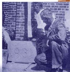
STEPHEN JAISLE PLACING CORNER STONE - 1931
