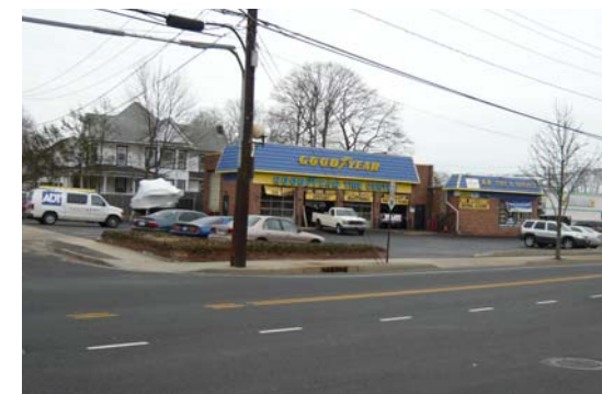
The Village has a number of chain-strip types of developments that includes gas stations, restaurants and convenience retailers. This type of development characterized by designs that are unresponsive to local architectural and aesthetic context is not compatible with the Village's aesthetic vision.
