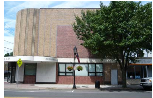
360 Main Street (former Farmingdale Movie Theater) is an excellent example of Art Deco architecture. While its adaptive reuse included an aluminum fenestration system, the building form and style remain mostly intact.
