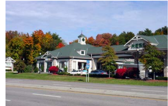
This Hess gas station located in Dutchess County is an example of a national chain incorporating locally responsive design elements into its building (desirable). The site is also attractively landscaped.
