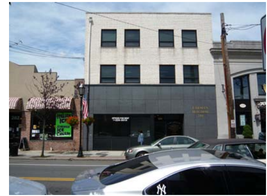
While attractive and constructed of quality materials, this façade retrofit presents a monolithic appearance, which does not contribute positively to the finer-grained appearance of a traditional Main Street. The building, one of the tallest on Main Street, could also be improved with a cornice or cap.
