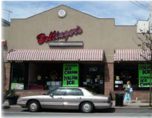
The condition of signage along Main Street varies. This unique sign actually compliments the building, but it is missing lenses in front of letters and the awning is tattered and sun-faded. The large green window posters are unnecessary and contribute to a cluttered appearance along the street and detract from the pedestrian experience.
