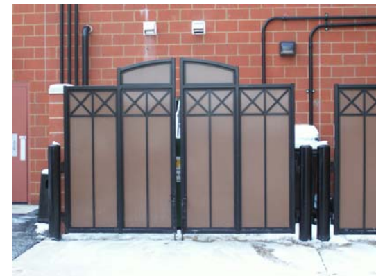
These nicely designed gates screen refuse containers and present an attractive architectural appearance.
