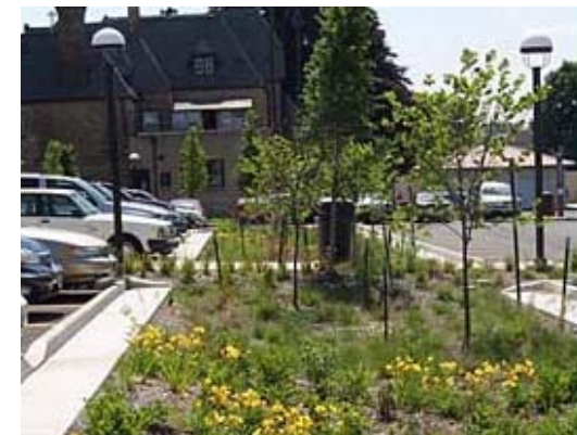
Parking areas can be designed to be more attractive and environmentally sensitive. Dividers and medians can be used to catch and filter hard surface run-off.
