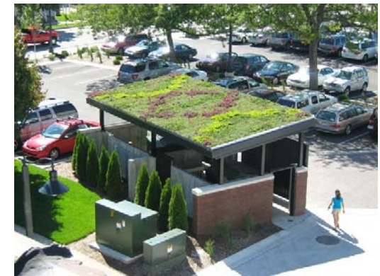
An exceptionally well designed refuse enclosure and parking lot in a typical corridor residential development.
