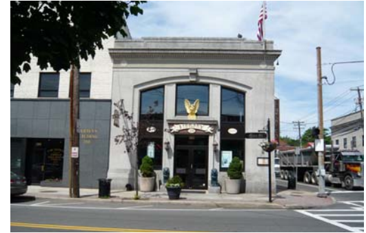
The Library Café: an excellent example of adaptive reuse, including signage, that respects the architectural heritage of the original historic building.
