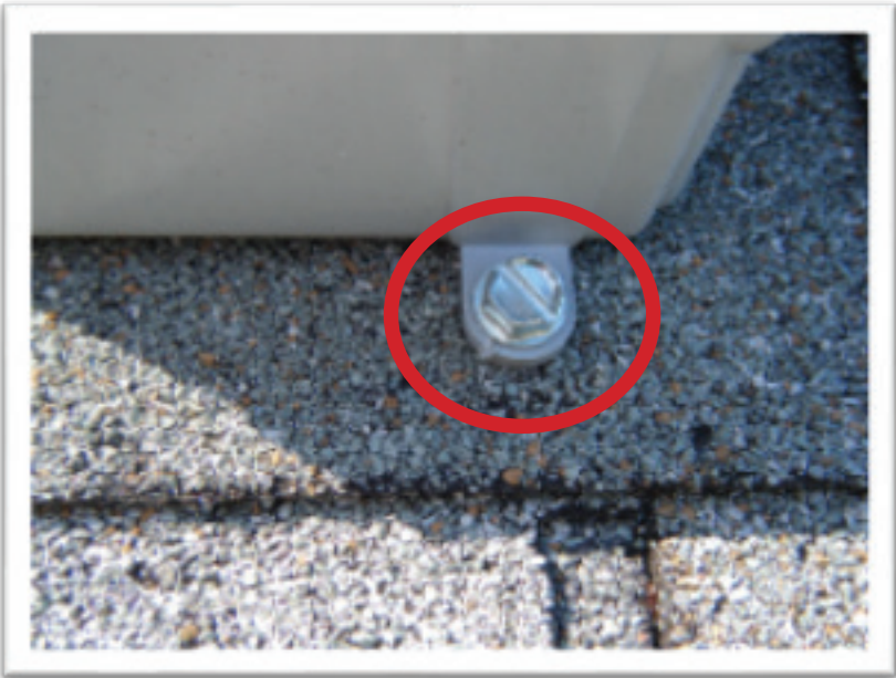
Photo D6: Roof penetrations and anchors not flashed: International Building Code 1503.2, International Residential Code 903.2.
