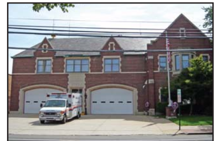
Village Hall/Fire Department
