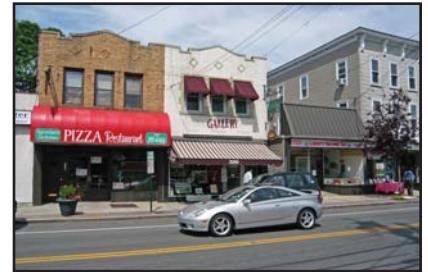
Retrofitted building along Main Street
