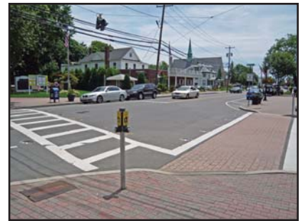
Pedestrian crosswalks near Village Hall
