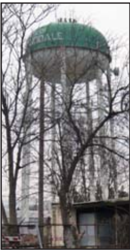
Water District Water Tower
