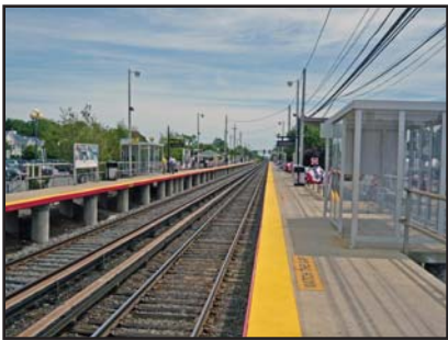
Farmingdale Long Island Rail Road Station
