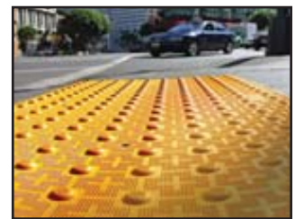
Tactile surface treatment
